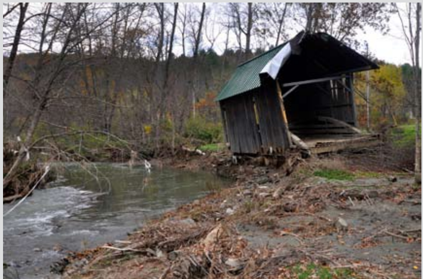
Flooding rains from Hurricane Irene destroyed roads and bridges throughout Vermont. The historic Bowers covered bridge (above), built in 1919, was lifted off its abutments and carried 200 feet downstream.
